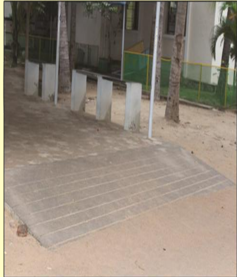
Ramp and Passage connecting Tarbes Block and Durier Block
